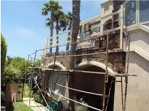
Before: Facade of 14 year-old custom coastal residence (Laguna Beach, CA) with severe damage due to improper waterproofing of parapet wall, etc.
