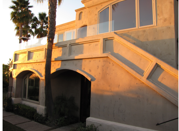
After: Facade of residence after renovations. CBCI repaired/replaced structural wood damage, stucco, windows, parapet wall, seamless glass wind screen, and waterproof deck.
