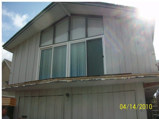
Before: Front of house after removing deteriorated railing from water-damaged deck
